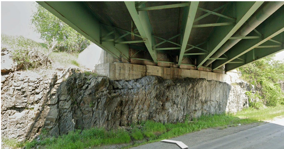
Photograph 2 – East abutment footing bearing on bedrock. Note presence of half casts from drillholes used as perimeter control during bedrock removal for the existing bridge.
