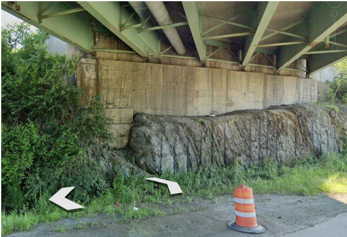
Photograph 1 – West abutment footing bearing on bedrock. Note presence of half casts from drillholes used as perimeter control during bedrock removal for the existing bridge. Note the variable top of bedrock surface.
